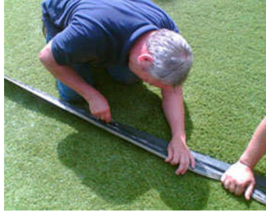
2. Trimming edge of grass prior to applying the glue
