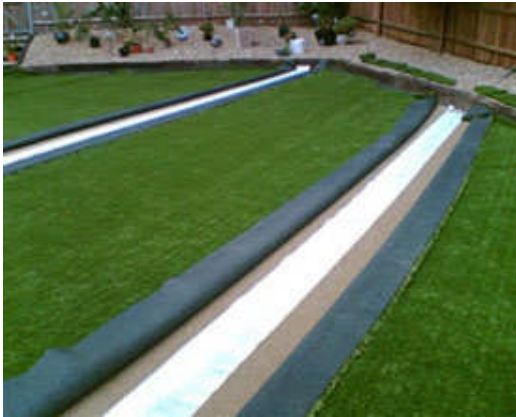
3. Jointing tape in place
